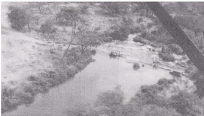
Above Aerial View - Ford crossing/concrete drift, one of the larger short term jobs surveyed, planned and designed.
