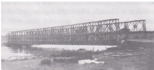
Left - a double/double bailey supported on bank grillage Below - more pictures of wet bailey bridges
