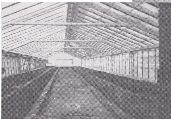
The second glasshouse under construction after a short 4 day electric welding course built with 2 inch second-hand galvanised pipe
