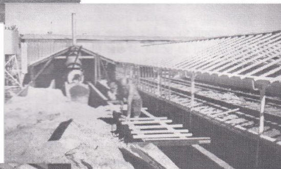
The second glasshouse under construction after a short 4 day electric welding course built with 2 inch second-hand galvanised pipe
