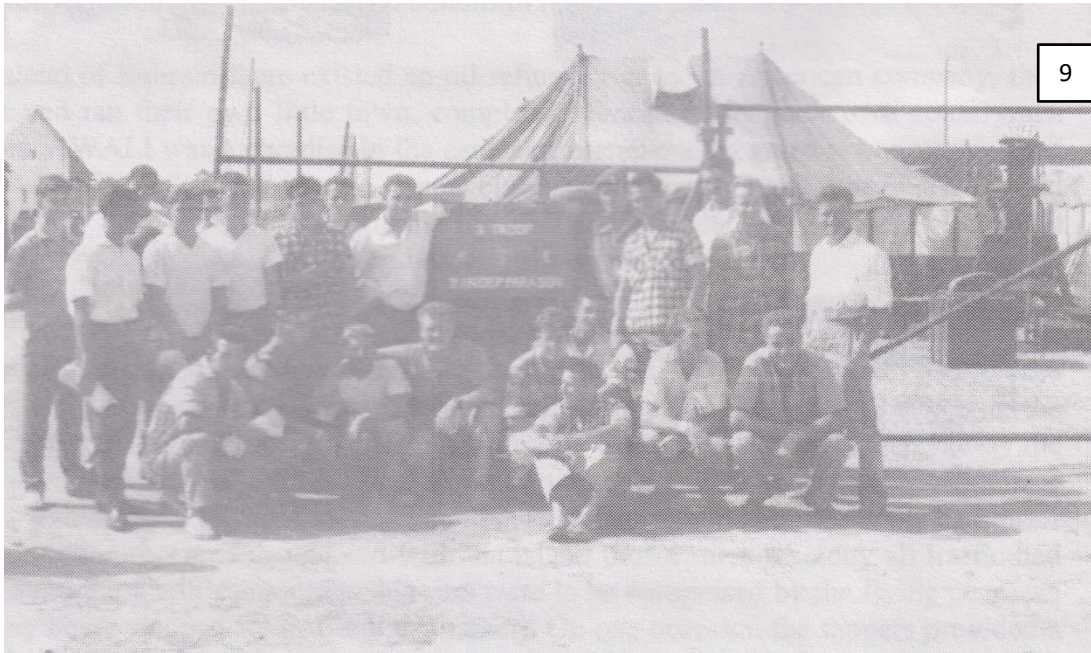
7. Internal cladding 8. One half of almost finished and furnished Twynham Hut 9. Construction crew within the confines of Jufair Naval Base 1961
