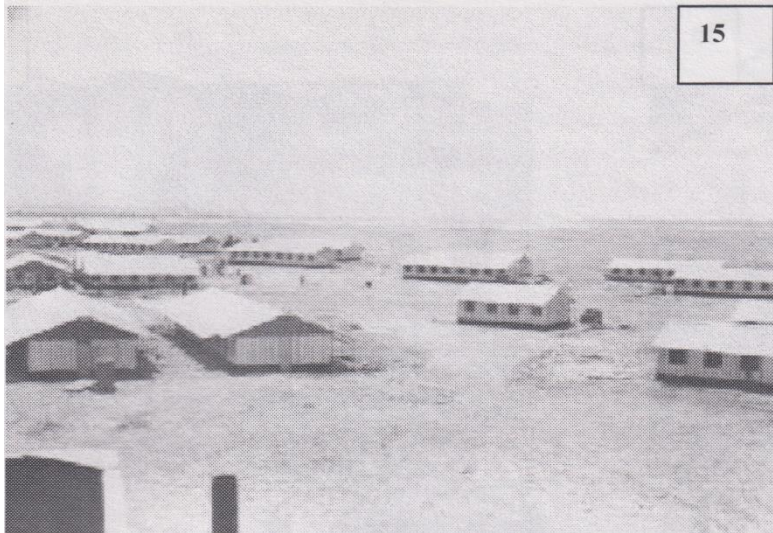
15. Huts nearing completion
