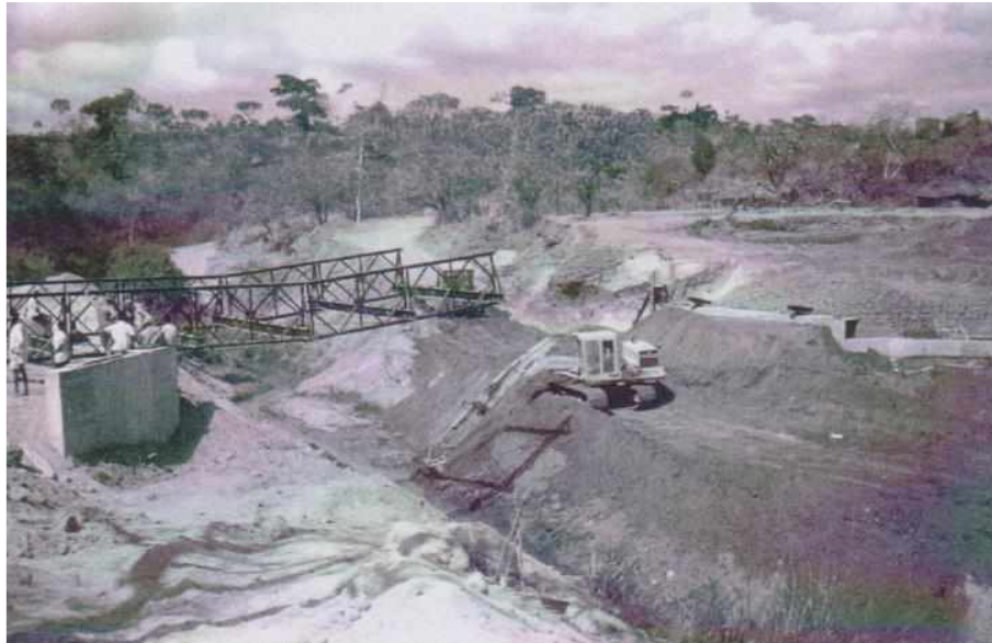
Construction of the Bailey Bridge launching nose
